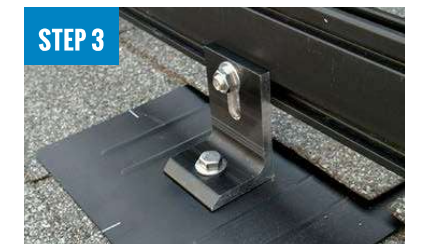
STEP 3 ATTACH L-FOOT TO RAIL
