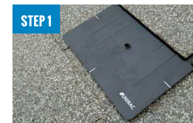
STEP 1 INSTALL FLASHKIT PRO FLASHING
