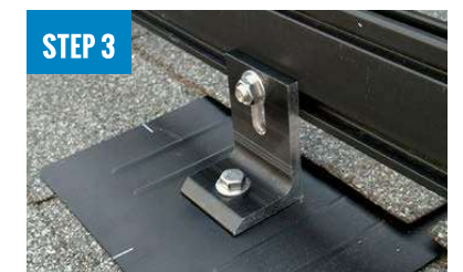
STEP 3 ATTACH L-FOOT TO RAIL
