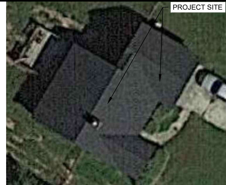
2 HOUSE PHOTO PV-1 SCALE: NTS
