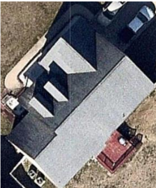
TOP VIEW OF BUILDING
