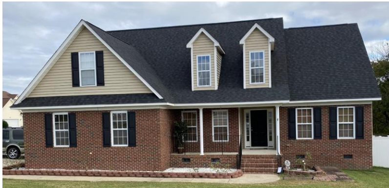
FRONT VIEW OF BUILDING
