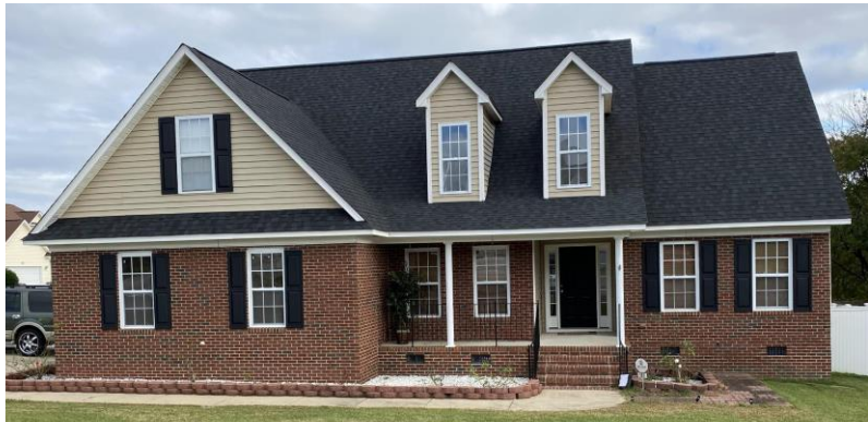
FRONT VIEW OF BUILDING
