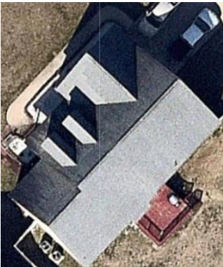
TOP VIEW OF BUILDING
