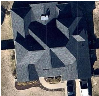
TOP VIEW OF BUILDING
