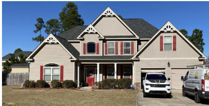
FRONT VIEW OF BUILDING
