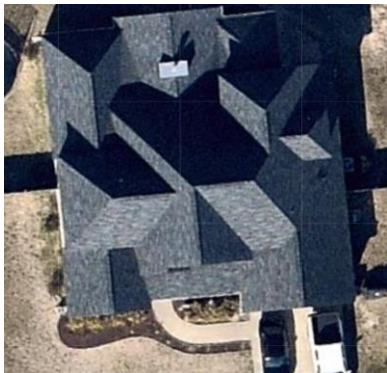
TOP VIEW OF BUILDING
