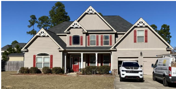
FRONT VIEW OF BUILDING
