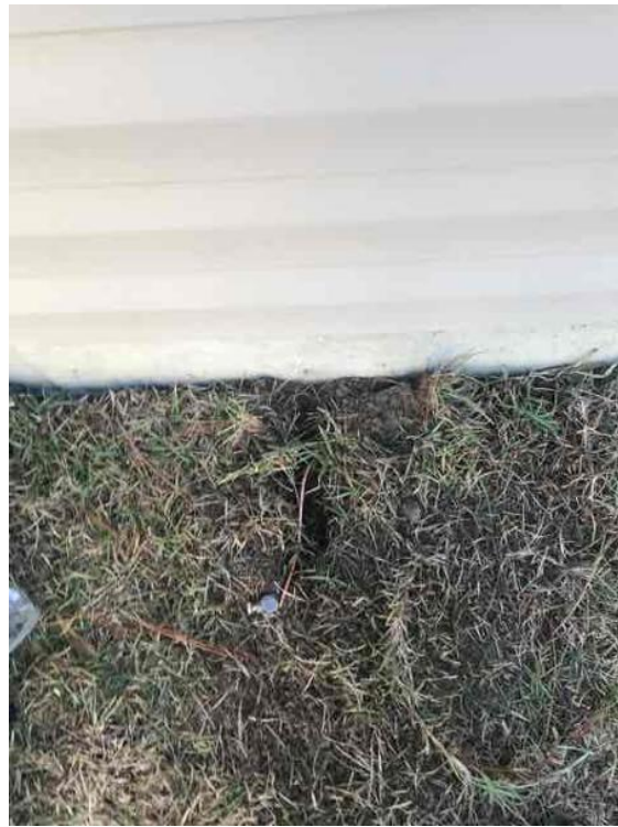
Roof/Array Information - Photo: Conduit Run
