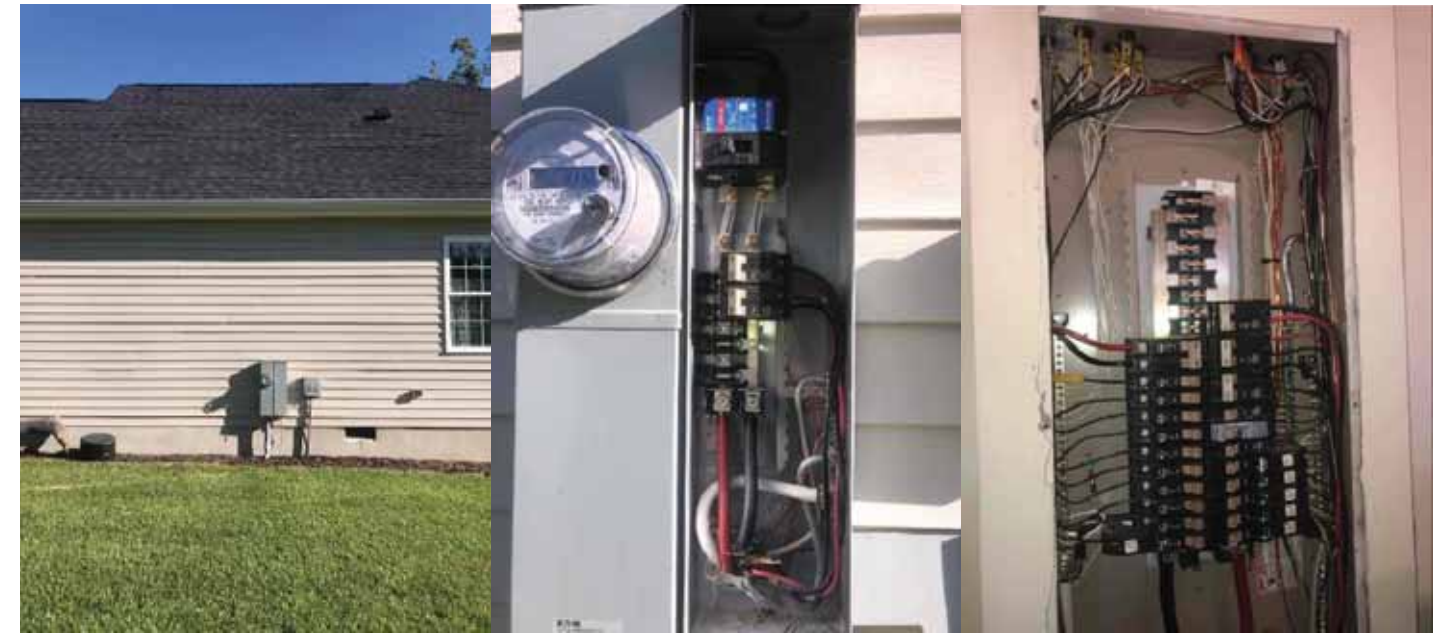
Utility Company: Duke Energy NC Permit Issuer: Harnett County
