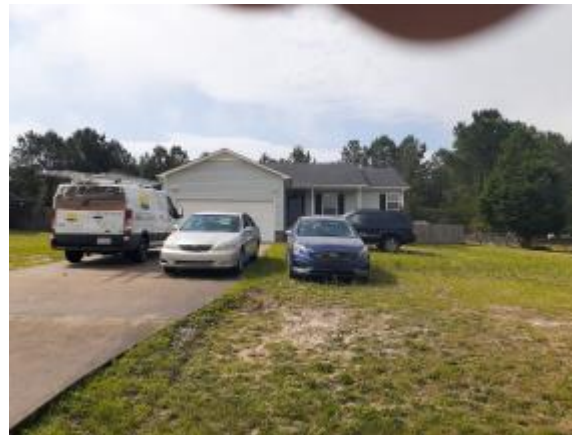
FRONT VIEW OF BUILDING
