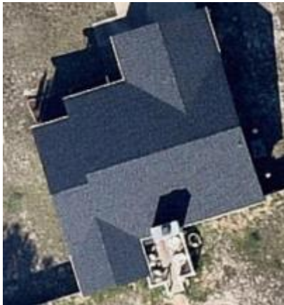
TOP VIEW OF BUILDING
