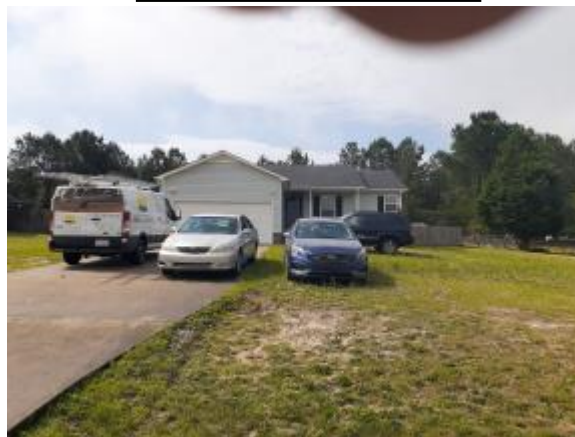
FRONT VIEW OF BUILDING
