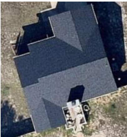
TOP VIEW OF BUILDING
