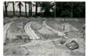
amy Repair SR1793 Pope RC
