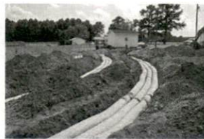
amy Repair SR1793 Pope RC
