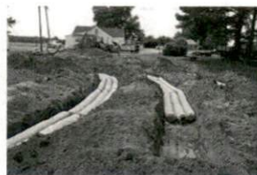
amy Repair SR1793 Pope RC
