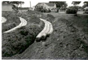
amy Repair SR1793 Pope RC
