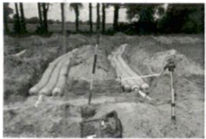
amy Repair SR1793 Pope RC
