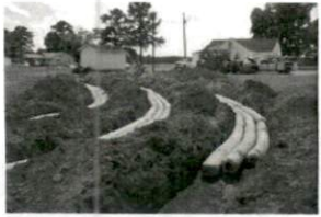
amy Repair SR1793 Pope RC
