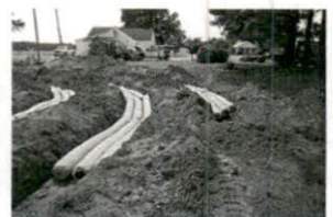
amy Repair SR1793 Pope RC
