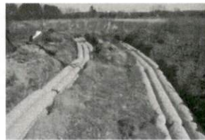
Jucas Repair 3-5-18 SR 1793 P
