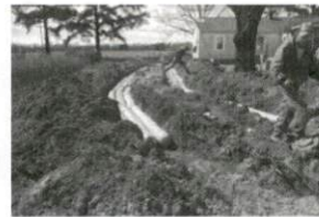
Jucas Repair 3-5-18 SR 1793 P
