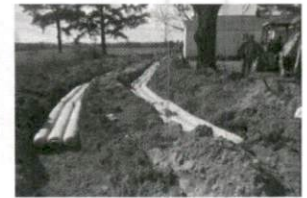
Jucas Repair 3-5-18 SR 1793 P
