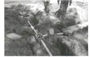
Jucas Repair 3-5-18 SR 1793 P
