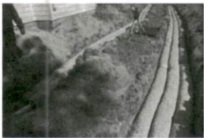
Jucas Repair 3-5-18 SR 1793 P
