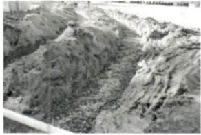
Repair 12-28-11 SR 1566 La
