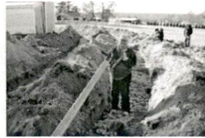
on Repair 12-28-11 SR 1566 L
