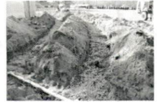
Repair 12-28-11 SR 1566 La
