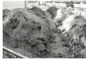
Repair 12-28-11 SR 1566 La
