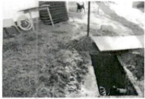
Repair 12-28-11 SR 1566 La
