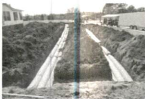
s Repair 5-1-17 SR 1712 Hob
