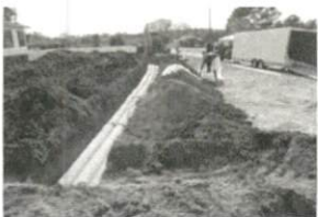
s Repair 5-1-17 SR 1712 Hob
