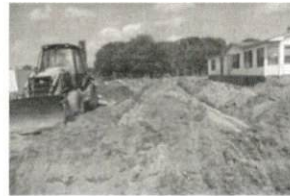
s Repair 5-1-17 SR 1712 Hob
