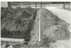
s Repair 5-1-17 SR 1712 Hob
