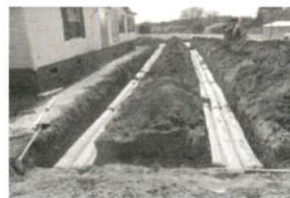
s Repair 5-1-17 SR 1712 Hob
