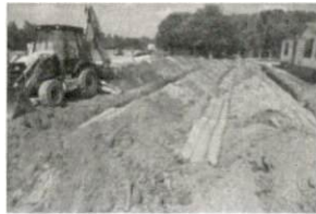
s Repair 5-1-17 SR 1712 Hob
