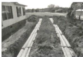
s Repair 5-1-17 SR 1712 Hob
