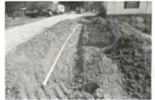
s Repair 5-1-17 SR 1712 Hob
