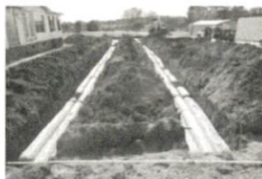
s Repair 5-1-17 SR 1712 Hob
