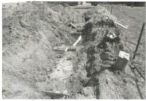
s Repair 5-1-17 SR 1712 Hob
