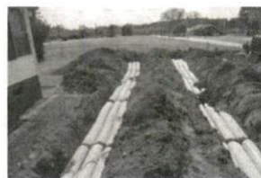
s Repair 5-1-17 SR 1712 Hob
