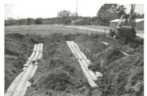
s Repair 5-1-17 SR 1712 Hob
