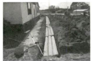
s Repair 5-1-17 SR 1712 Hob
