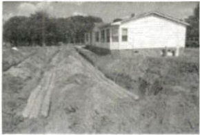
s Repair 5-1-17 SR 1712 Hob
