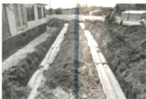
s Repair 5-1-17 SR 1712 Hob
