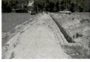
1 Repair 9-27-17 SR1403 Kipli
