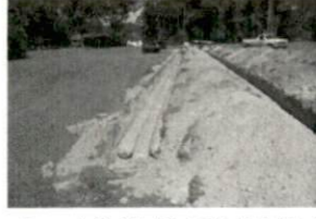
1 Repair 9-27-17 SR1403 Kipli
