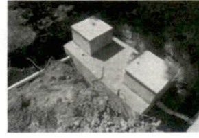
1 Repair 9-27-17 SR1403 Kiplir
