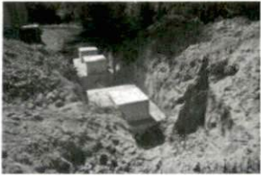
1 Repair 9-27-17 SR1403 Kiplir
