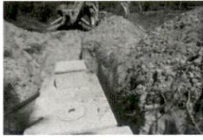
1 Repair 9-27-17 SR1403 Kiplir
