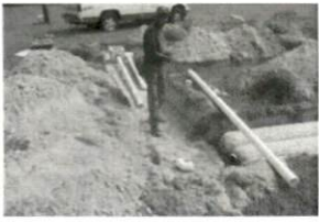
1 Repair 9-27-17 SR1403 Kipli
