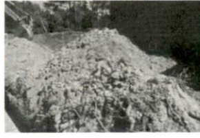
1 Repair 9-27-17 SR1403 Kiplir
