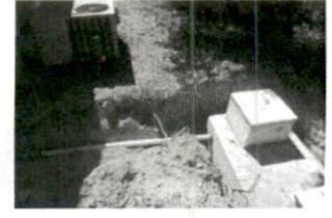
1 Repair 9-27-17 SR1403 Kiplir
