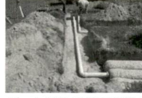
1 Repair 9-27-17 SR1403 Kipli
