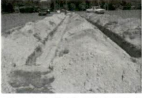
1 Repair 9-27-17 SR1403 Kipli
