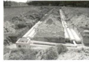
1 Repair 9-27-17 SR1403 Kipli
