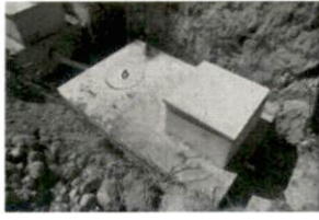
1 Repair 9-27-17 SR1403 Kiplir
