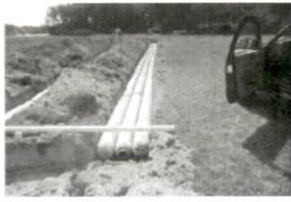
1 Repair 9-27-17 SR1403 Kipli
