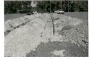
1 Repair 9-27-17 SR1403 Kipli
