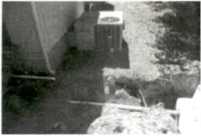
1 Repair 9-27-17 SR1403 Kiplir
