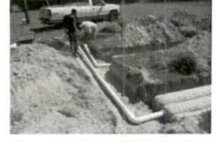
1 Repair 9-27-17 SR1403 Kiplir
