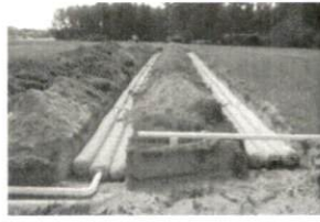
1 Repair 9-27-17 SR1403 Kipli
