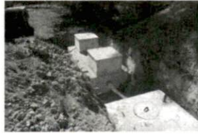
1 Repair 9-27-17 SR1403 Kiplir
