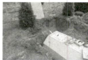
Jorris Tank Replace Hwy 27 8
