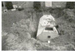
Jorris Tank Replace Hwy 27 8
