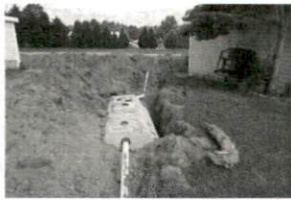
ngdon Repair 6-8-18 SR1532
