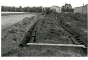
ngdon Repair 6-8-18 SR1532
