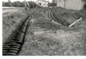
ngdon Repair 6-8-18 SR1532
