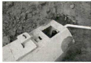
ngdon Repair 6-8-18 SR1532
