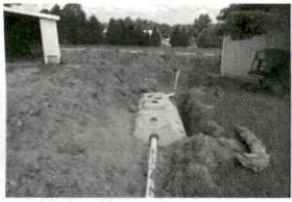
ngdon Repair 6-8-18 SR1532
