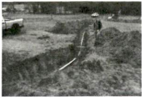
I Davies Repair HWY 27 12-8-
