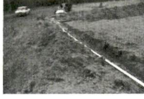
I Davies Repair HWY 27 12-8-
