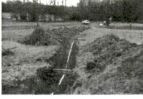
I Davies Repair HWY 27 12-8-
