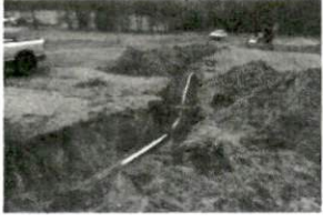
I Davies Repair HWY 27 12-8-
