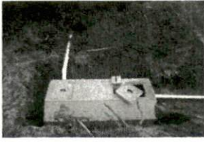
Davies Repair HWY 27 12-8-
