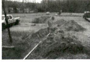
Davies Repair HWY 27 12-8-
