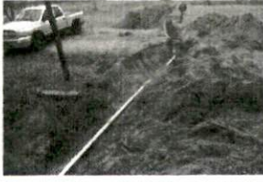
Davies Repair HWY 27 12-8-
