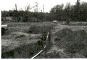
I Davies Repair HWY 27 12-8-
