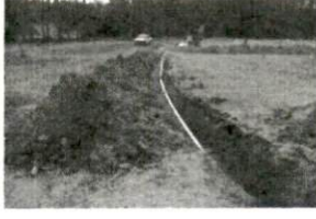
I Davies Repair HWY 27 12-8-
