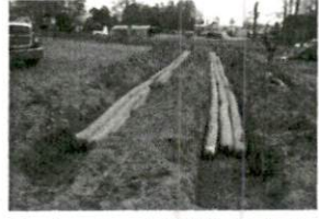
Davies Repair HWY 27 12-8-
