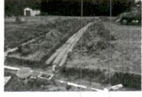
Davies Repair HWY 27 12-8-
