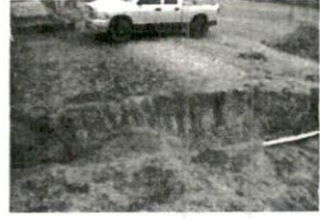
I Davies Repair HWY 27 12-8-
