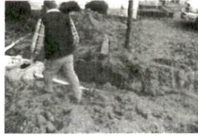
I Davies Repair HWY 27 12-8-
