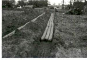
Davies Repair HWY 27 12-8-
