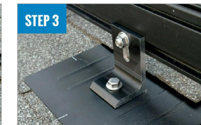
ATTACH L-FOOT TO RAIL
