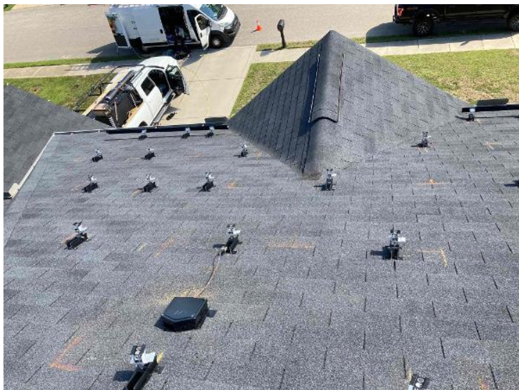
Module Installation / Ready for Modules (All rail-less parts required to land modules complete)
