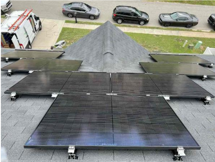
Module Installation / Close Up of Flashkit Slider Complete
