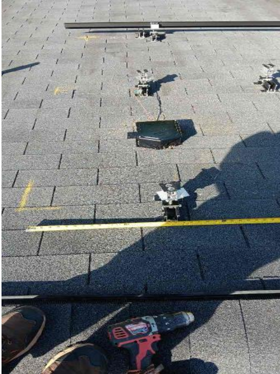
Module Installation / Ready for Modules (All rail-less parts required to land modules complete)
