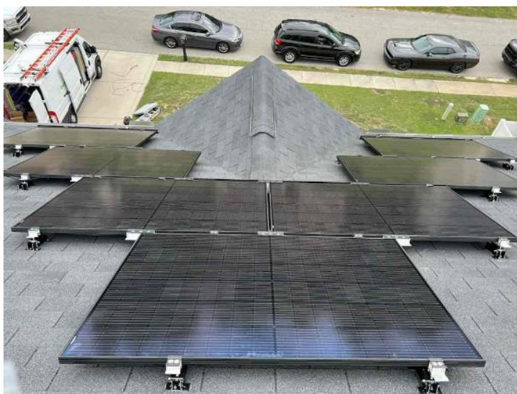
Module Installation / Module Gapping: Tape Measure showing 3/8" - 1" Gap
