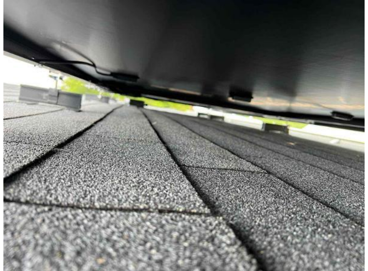
Module Installation / Wire management Under the Array (1 photo per row of modules per array)
