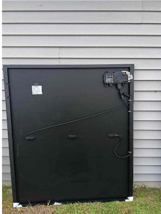
Module Installation / Optimizer + MLPE Mount
