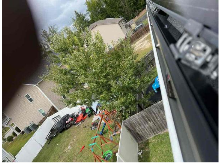
Module Installation / Close Up of Trimrail Splice + Trimrail Clip + Trimrail Roof Attachment Complete
