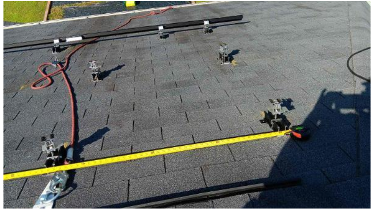
Module Installation / Ready for Modules (All rail-less parts required to land modules complete)
