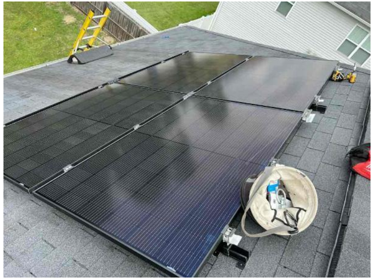
Module Installation / Close Up of 6.5" Splice Installed
