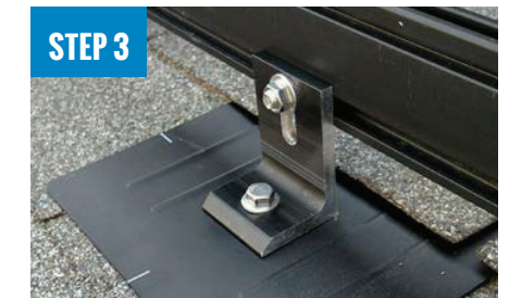
STEP 3 ATTACH L-FOOT TO RAIL
