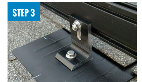
STEP 3 ATTACH L-FOOT TO RAIL
