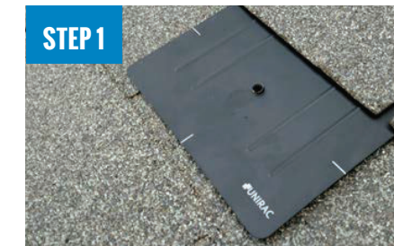
STEP 1 INSTALL FLASHKIT PRO FLASHING
