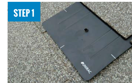
STEP 1 INSTALL FLASHKIT PRO FLASHING
