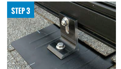
STEP 3 ATTACH L-FOOT TO RAIL
