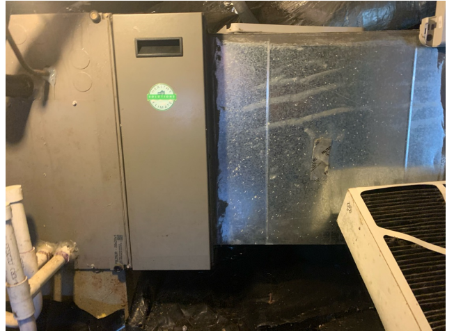
Photos of Existing Indoor System to be Removed (6 of 8)
