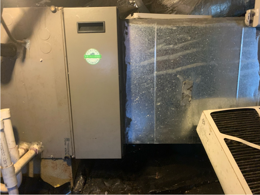
Indoor Modifications Picture with Mark up (7 of 8)
