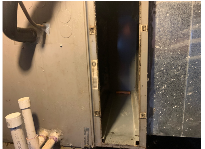
Photos of Existing Indoor System to be Removed (4 of 8)
