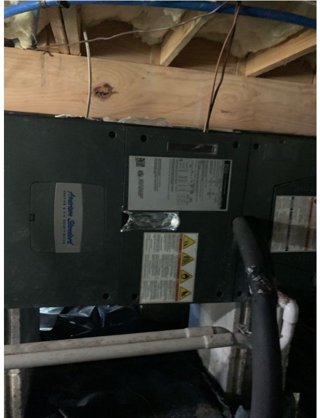
Photos of Existing Indoor System to be Removed (4 of 4)
