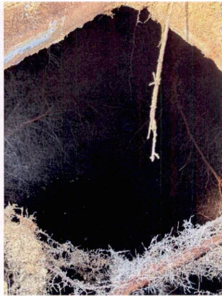
Root infiltration of inlet side
