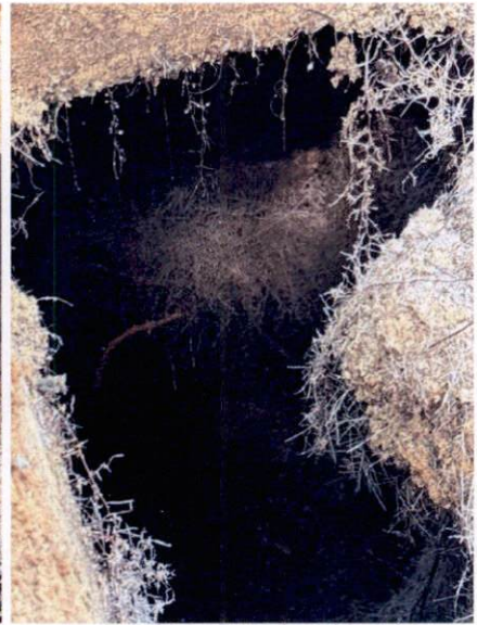
Root infiltration of outlet side
