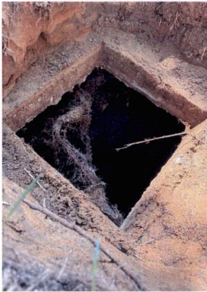
Root infiltration of inlet side of tank
