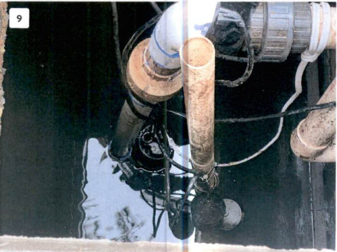
View of Pump and Alarm Floats
