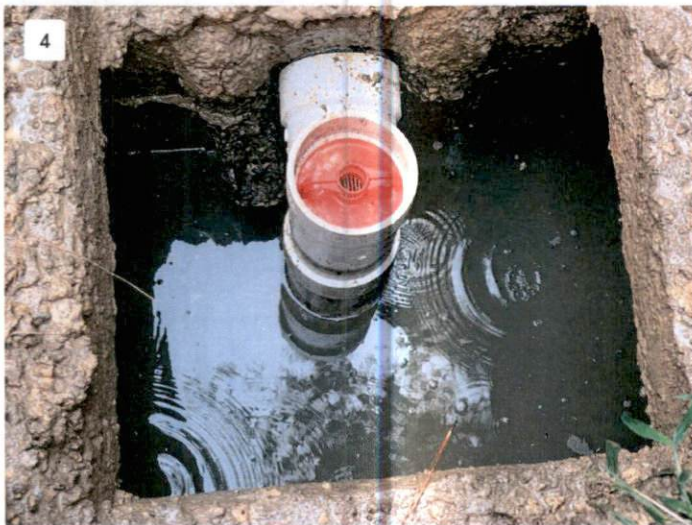
View of Septic Tank Outlet Tee
