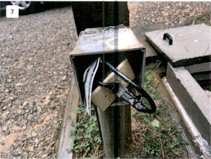
View of Inside of Control Panel, Control Panel Missing Cover Plate
