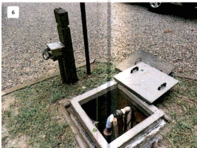
View of Location of Pump Tank Riser and Control Panel
