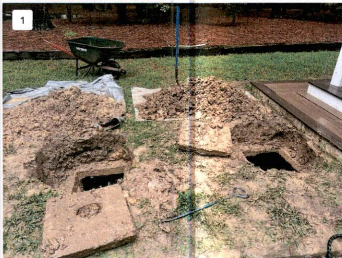
View of Location of Septic Tank Inlet and Outlet Lids
