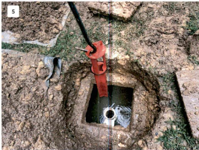
View of Clean Outlet Tee Filter
