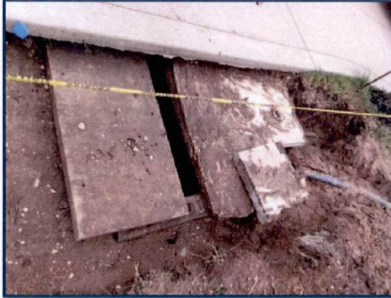
P7. Outlet End Slab Corner Cut Out
