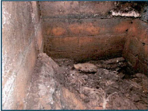
P19. Soil & Solid Waste In Septic Tank
