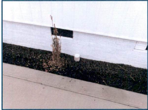
P4. Cleanout With Glued Test Cap
