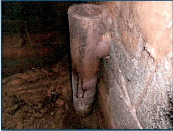
P19. Soil & Solid Waste In Septic Tank
