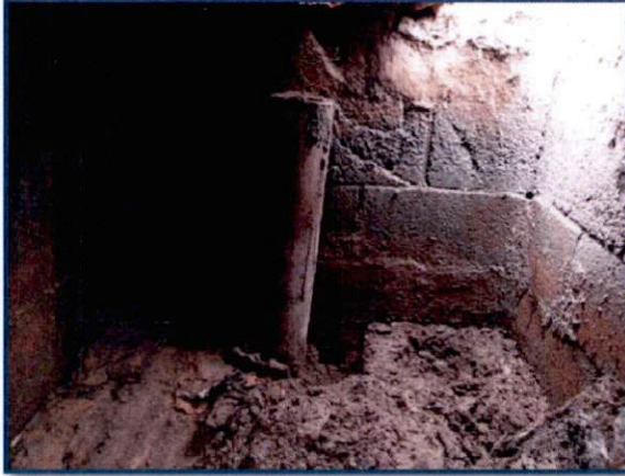
P15. Soil, Solid Waste, & Slab In Tank
