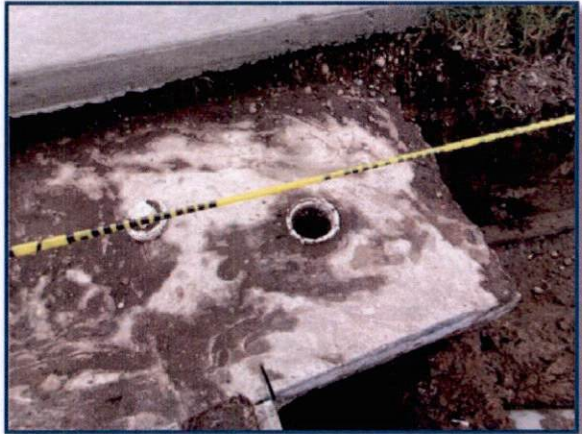
P8. Cleanout Installed In Outlet Slab
