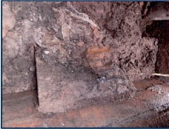
P15. Soil, Solid Waste, & Slab In Tank
