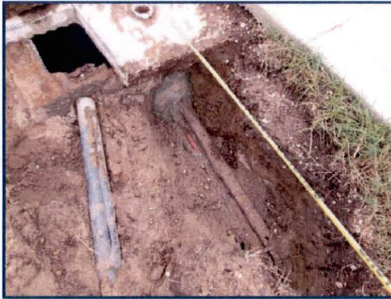
P23. Transition from Cast Iron To ABS
