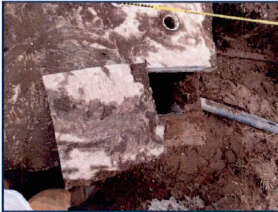
P7. Outlet End Slab Corner Cut Out
