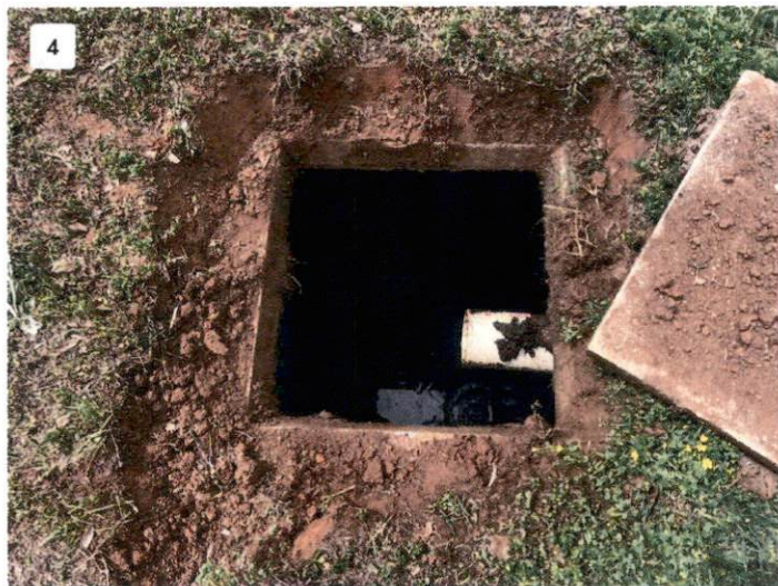
View of Septic Tank Inlet End
