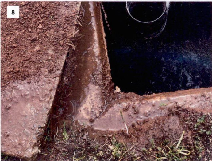
Crack at Outlet Lid Opening
