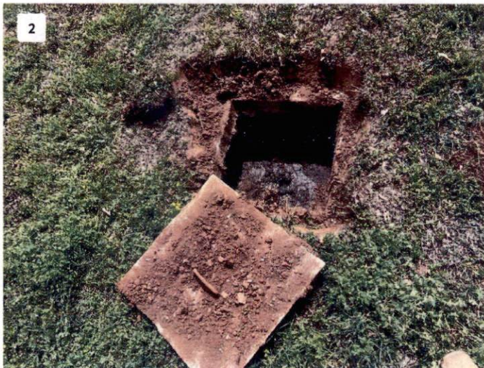
View of Septic Tank Inlet End
