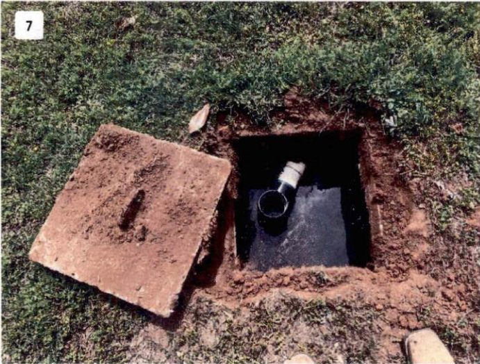
View of Septic Tank Outlet End
