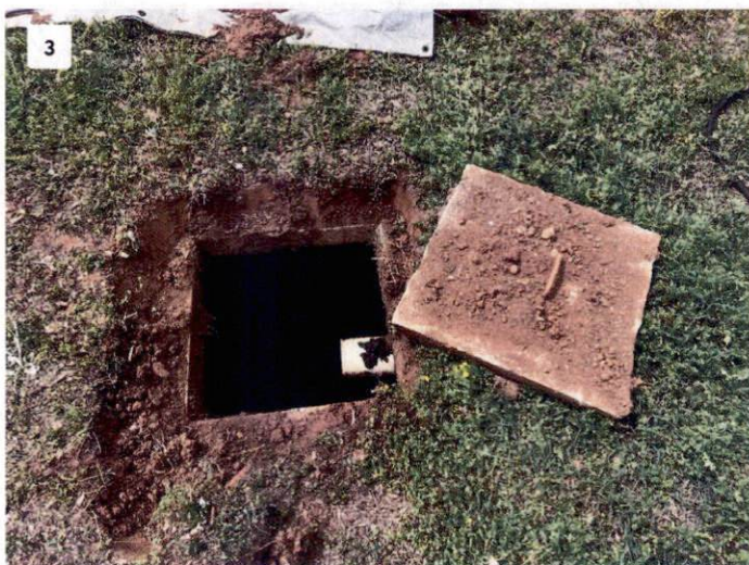
View of Septic Tank Inlet End
