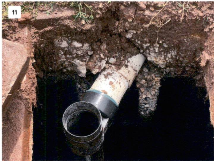
View of Septic Tank Outlet End
