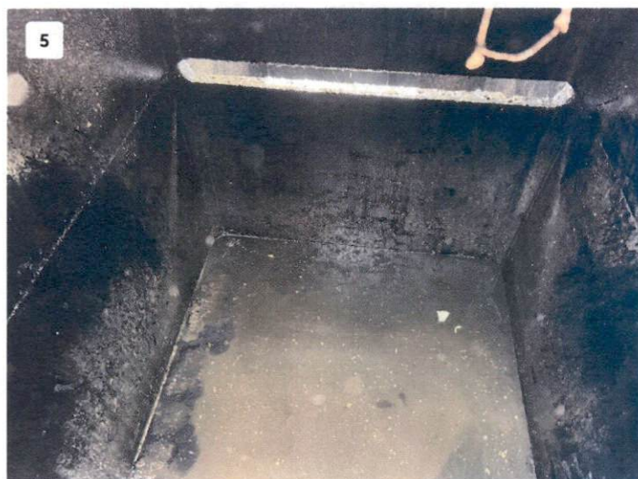
View of Baffle Wall
