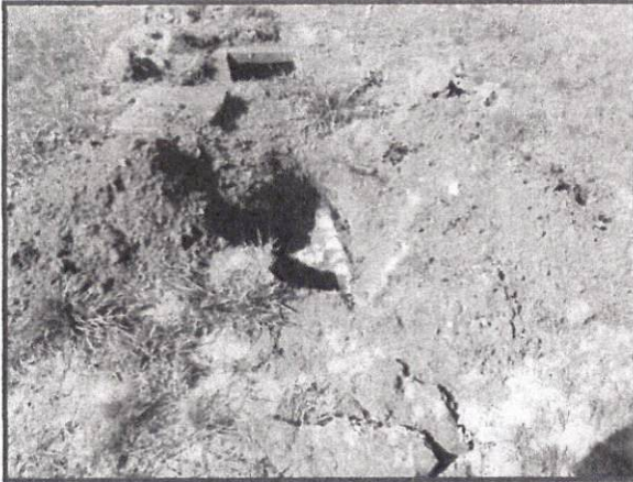
P11. Outlet Lid Cracked From Deterioration
