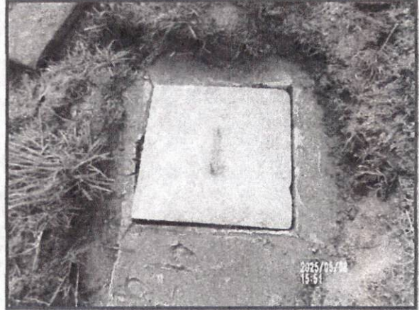
P12. Outlet Lid Replaced
