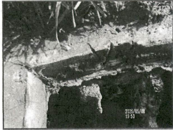
P16. Outlet End Wall Warped
