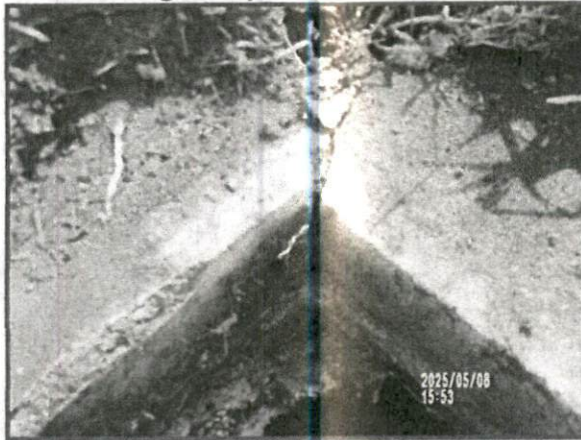
P15. Cracking In Top of Tank
