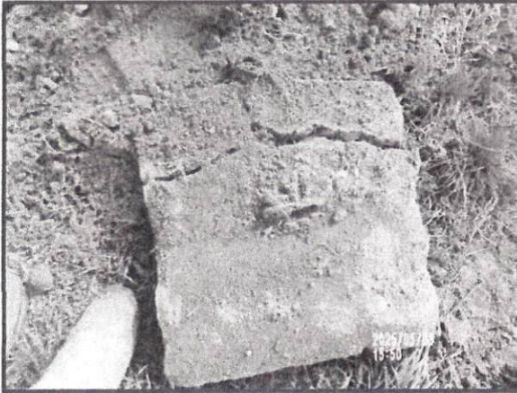
P11. Outlet Lid Cracked From Deterioration
