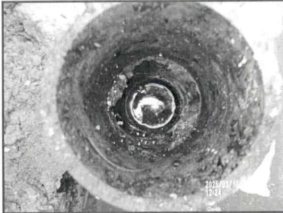
P15. Septic Tank Outlet Tee Not Secured
