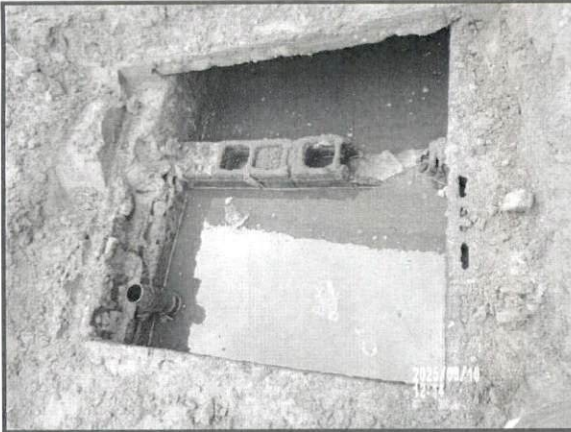
P7. Baffle Wall Damaged
