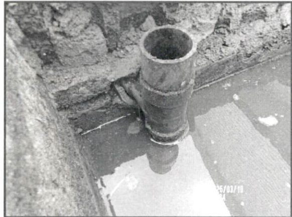
P12. Septic Tank Outlet Tee
