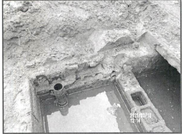
P8. Septic Tank Inlet Pipes
