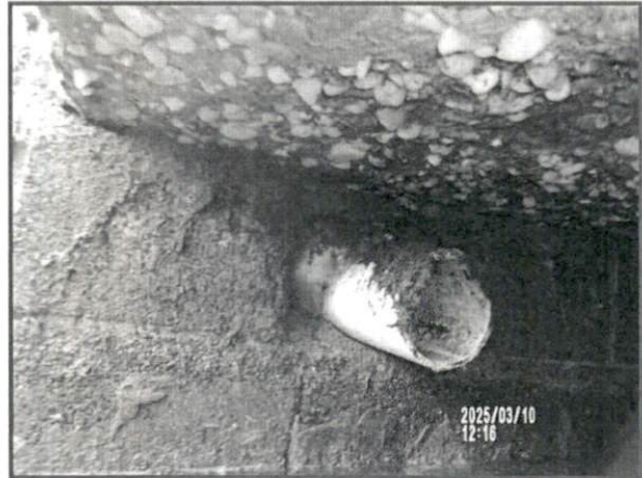
P12. Septic Tank Outlet Tee
