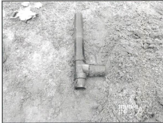
P15. Septic Tank Outlet Tee Not Secured
