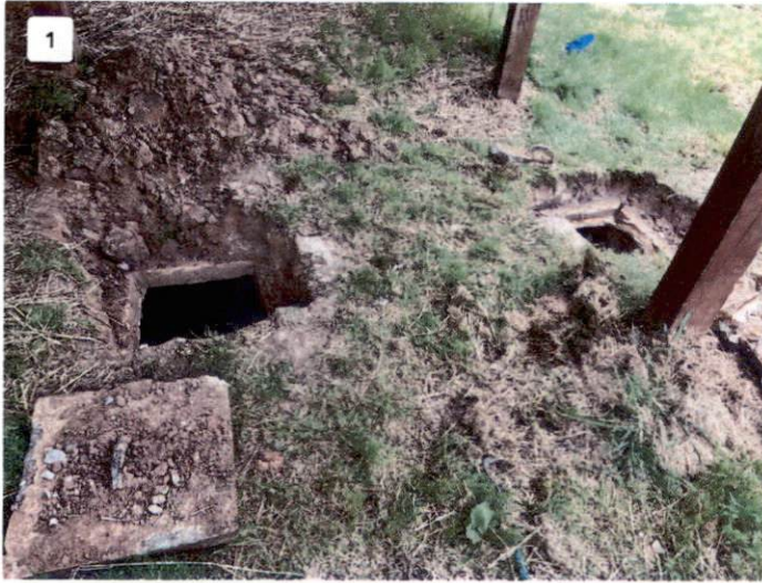
View of Location of Septic Tank Inlet and Outlet Lids
