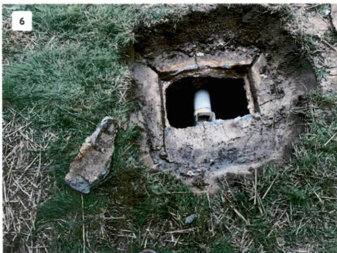
View of Septic Tank Outlet End
