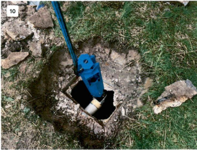
View of Clean Outlet Tee Filter
