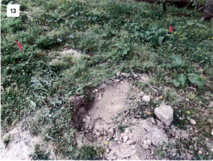
View of Location of Distribution Box
