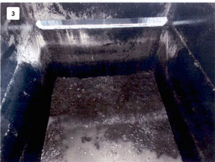
View of Inlet Compartment After Pumping of Tank
