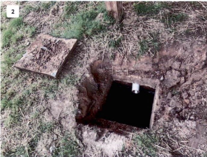
View of Septic Tank Inlet End
