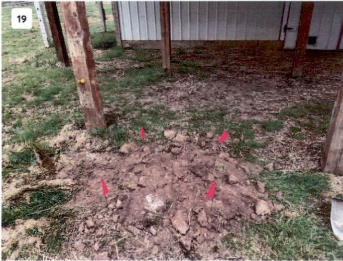
Excavations Filled and Site Cleaned
