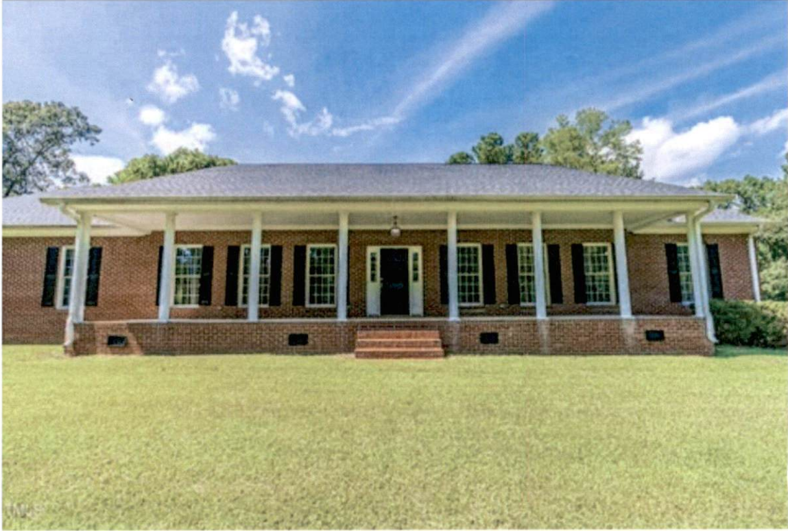
Inspection at current house
