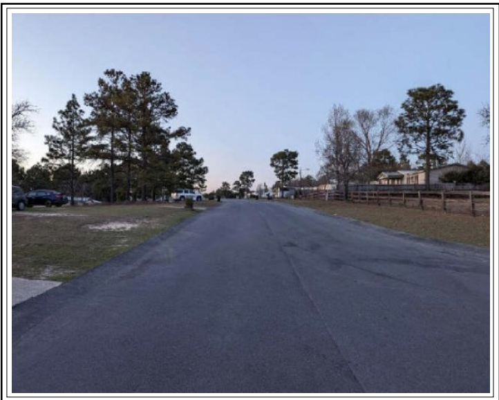
ADDITIONAL STREET SCENE
