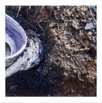
Precast wall or sanitary tee present / in-tact? (older tanks may have a concrete wall at the outlet that is prone to deterioration)
