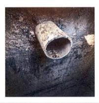
Inlet pipe above static water level? (an inlet pipe below the water level may cause a back up in the sewer line)
