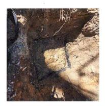
"At the time of inspection the water level was noted to be above both the inlet and outlet pipes and the dispersal field was not accepting any liquids."
