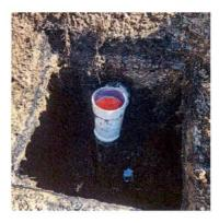
Is there an outlet filter present and needs cleaning? (newer tanks have an outlet filter that needs to be cleaned annually)
