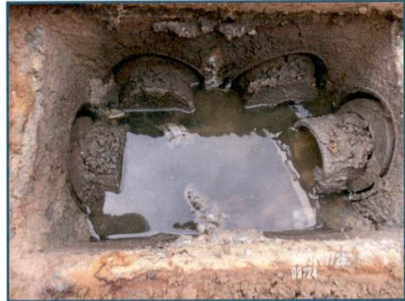
P26. Distribution Box—Before Flow Test
