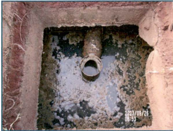
P21. Septic Tank Outlet Water Level
