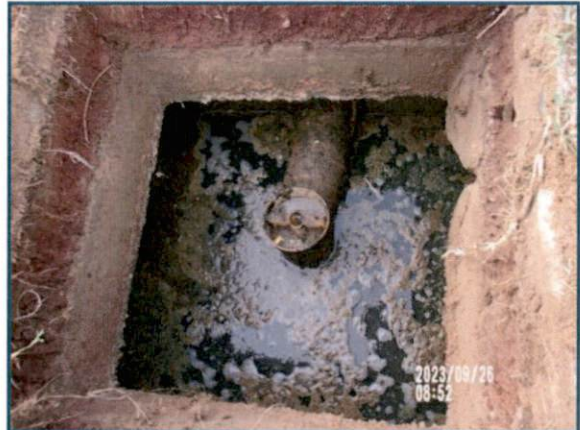
P14. Septic Tank Outlet Filter Tee
