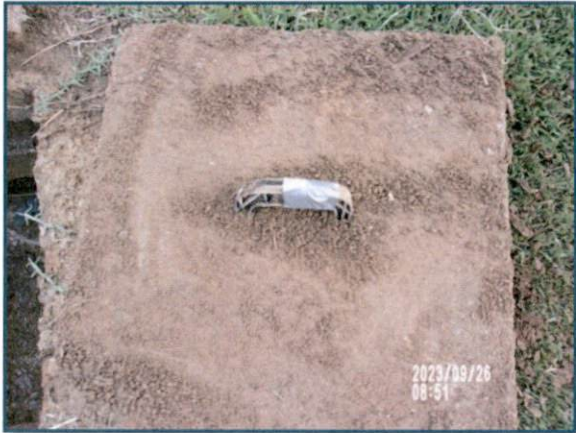
P5. Septic Tank Inlet Lid—Handle Broken
