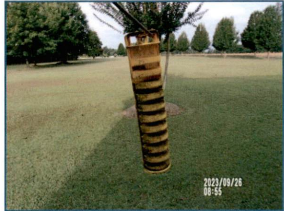
P22. Septic Tank Outlet Filter—Cleaned
