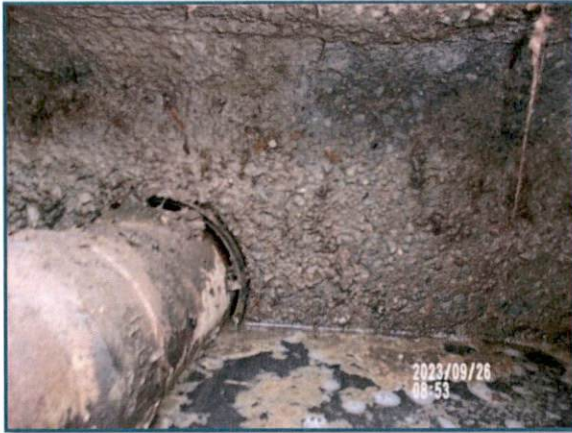
P21. Septic Tank Outlet Water Level
