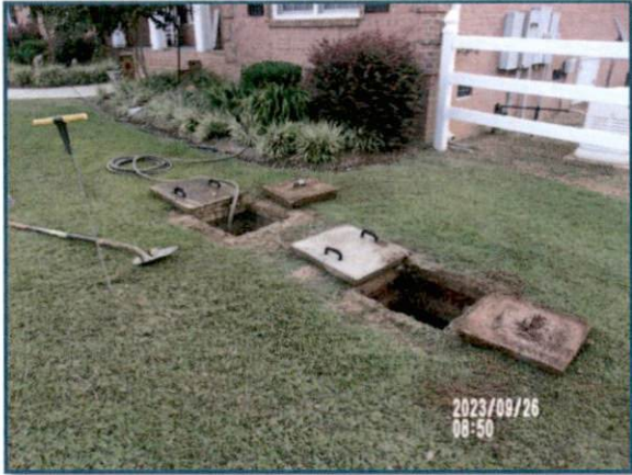
P5. Septic Tank Inlet Lid—Handle Broken
