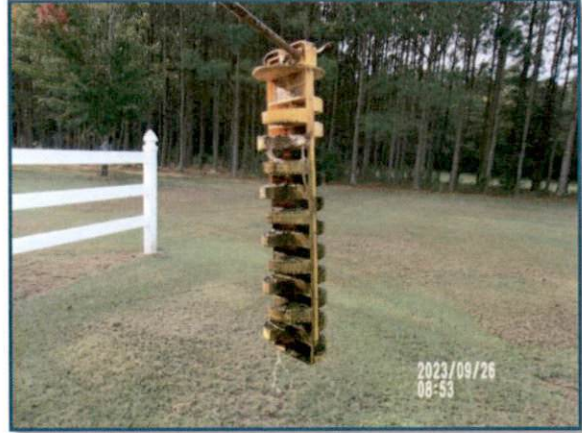
P22. Septic Tank Outlet Filter—Cleaned
