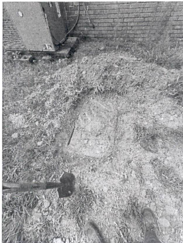
Figure 2 Located and dug up the septic tank lid
