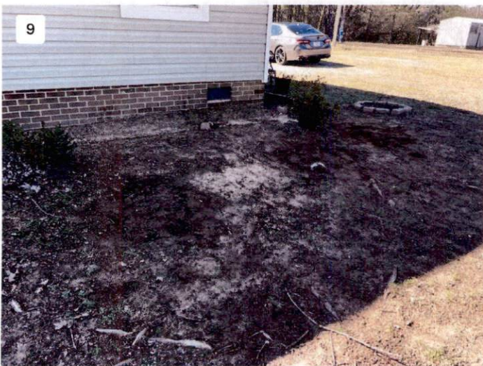
Excavations Filled and Site Cleaned
