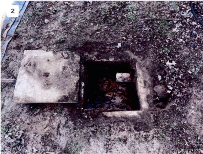
View of Septic Tank Inlet End
