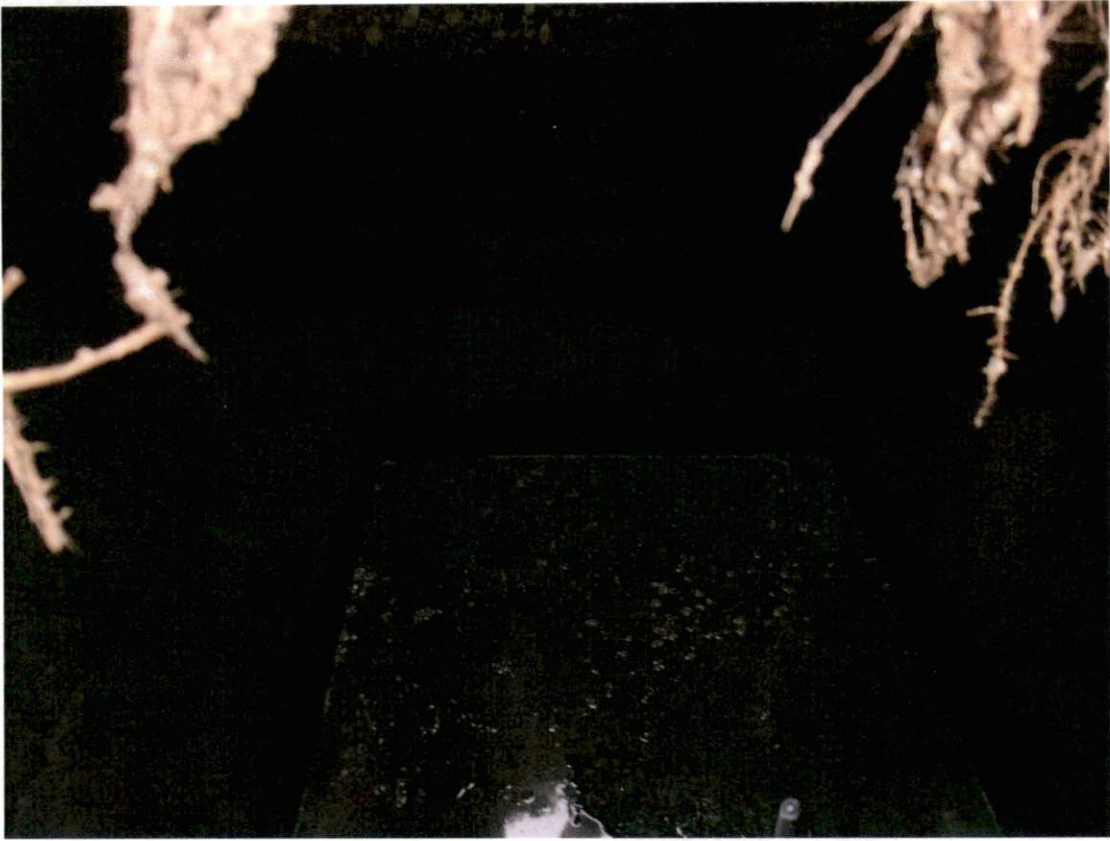
Inlet Compartment After Pumping
