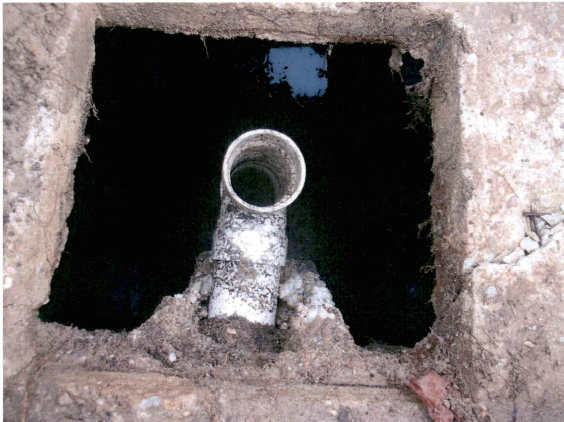
Outlet Compartment After Pumping
