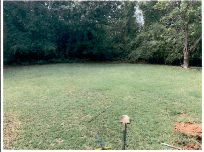
Suspected area of drain field
