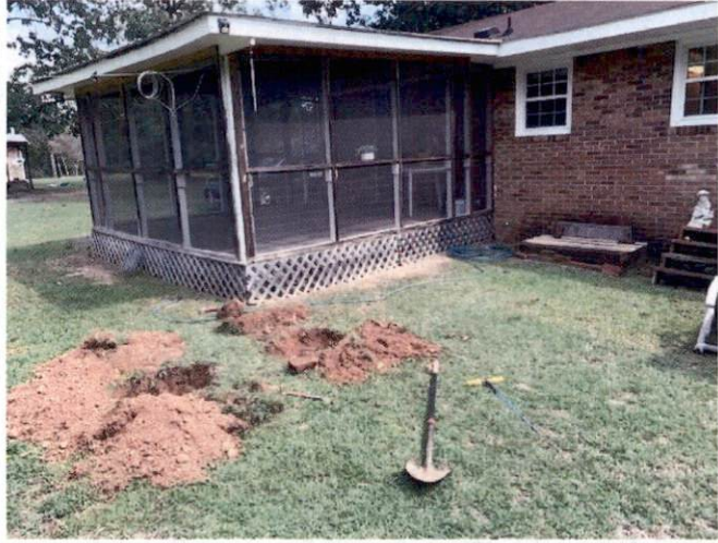
Septic tank location shown.
