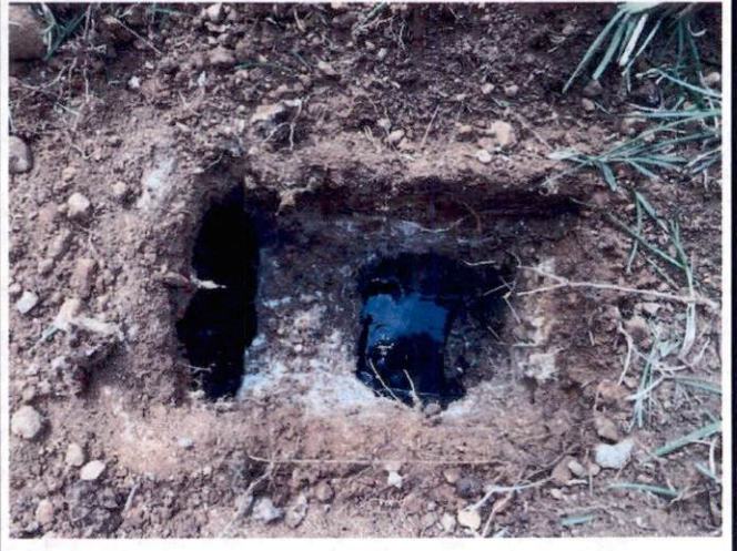
Outlet side of septic tank shown open for inspection
