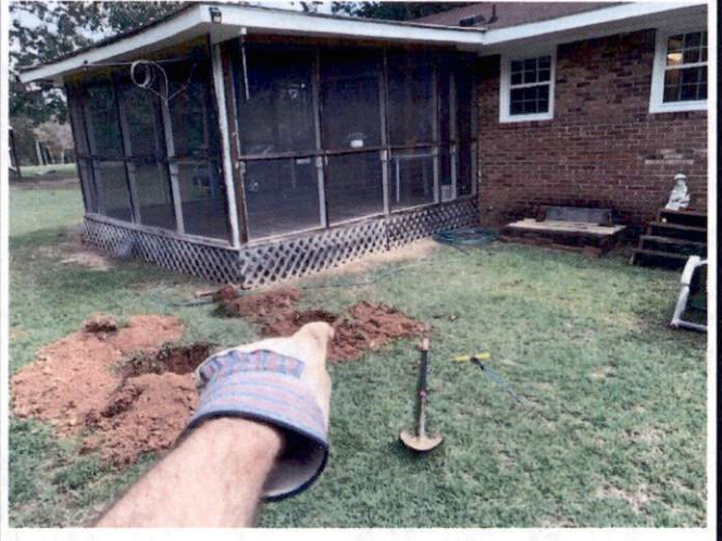
Outlet side of septic tank location shown
