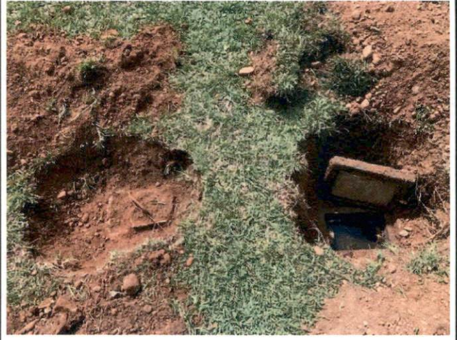
Location of distribution box shown behind septic tank
