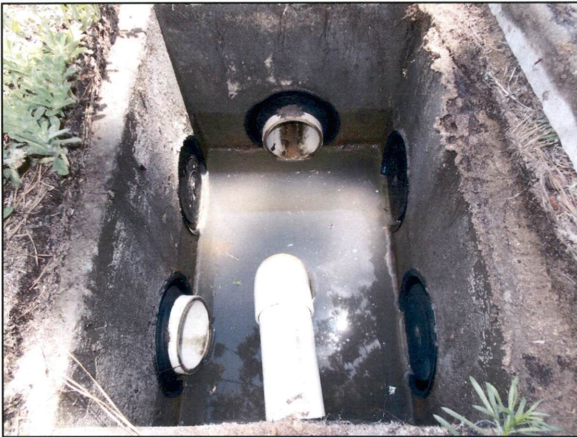
Example of Distribution Box with two (2) Lines:
