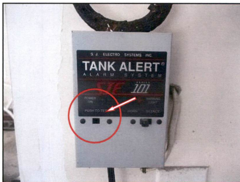
Example of Alarm (Test Switch):
