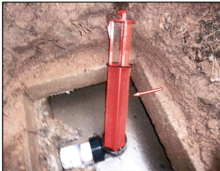
Example of Retro-fitted with PVC Sanitary Tee with Effluent Strainer:
