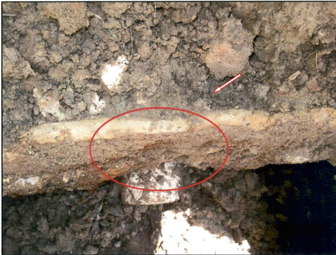
Outlet End Wall:
