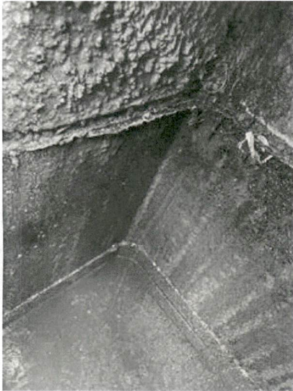
Septic Tank Walls
