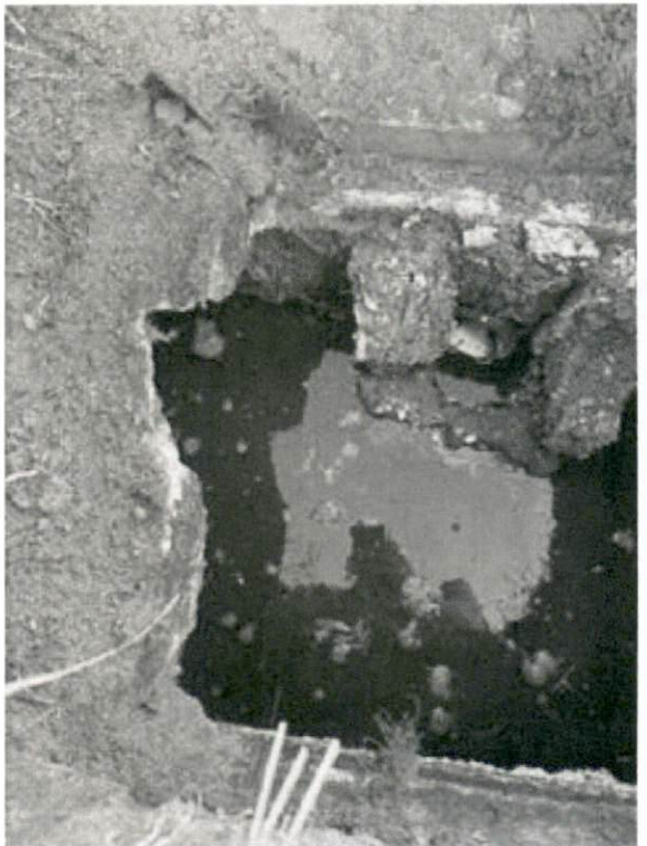
Outlet Side Before Pumping
