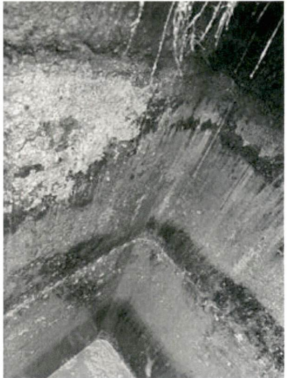
Septic Tank Walls
