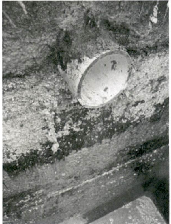
Inlet Sewer Line
