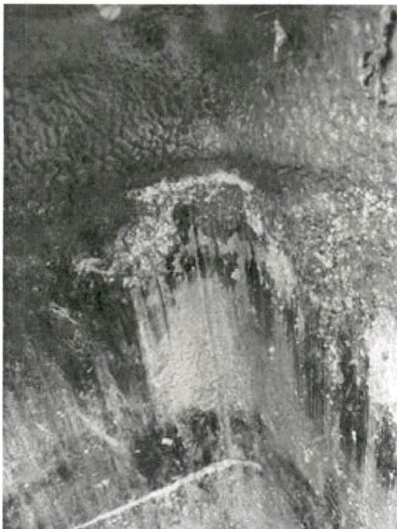
Septic Tank Walls
