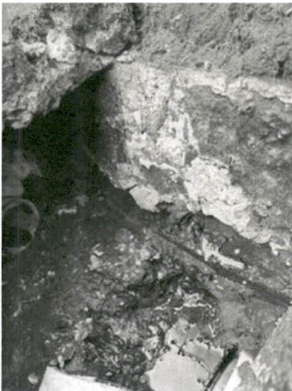
Inside Distribution Box
