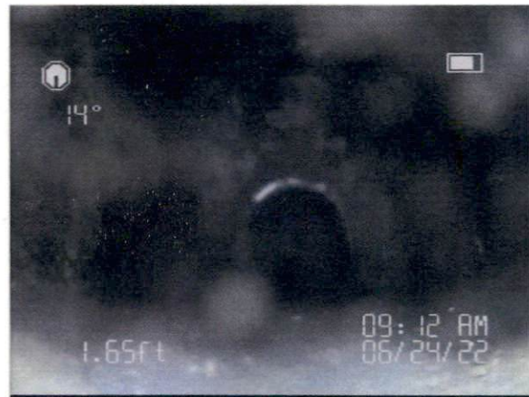
D-Box signs of Deterioration
