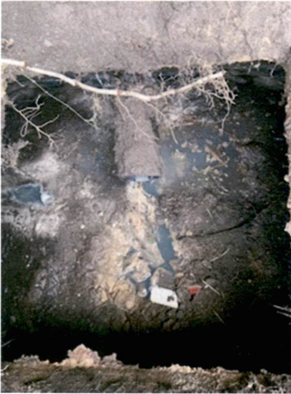
Inlet Side Before Pumping
