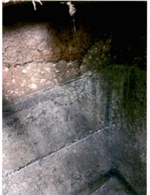
Septic Tank Walls
