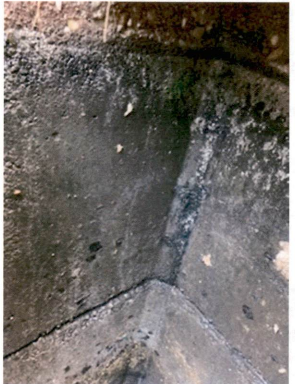
Septic Tank Walls
