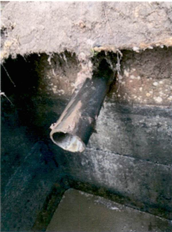
Inlet Sewer Line
