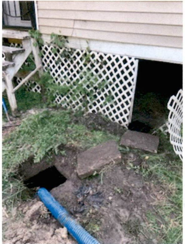
Septic Tank Location (Under the Home)
