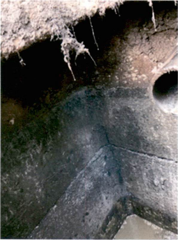
Septic Tank Walls
