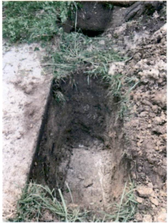
Distribution Box Location
