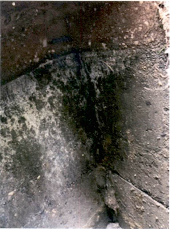
Septic Tank Walls
