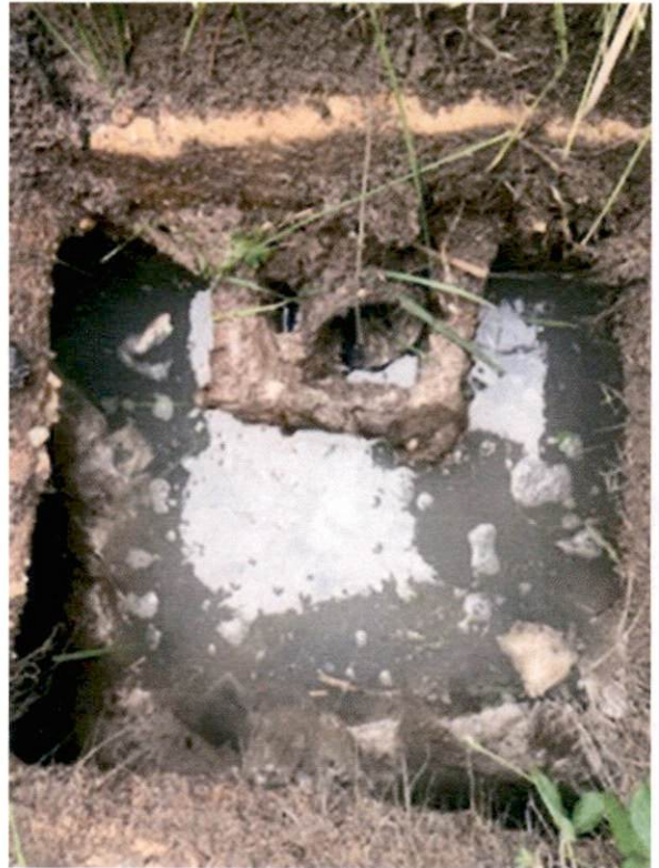
Outlet Side Before Pumping
