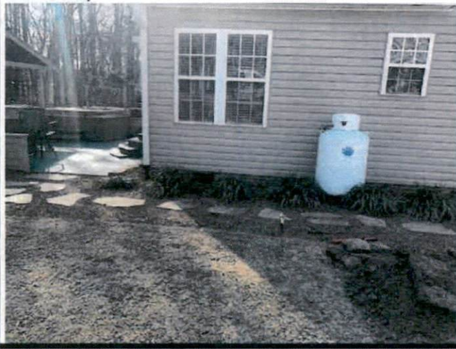
Area of drain field (Addition noted as being over top of drain field)
