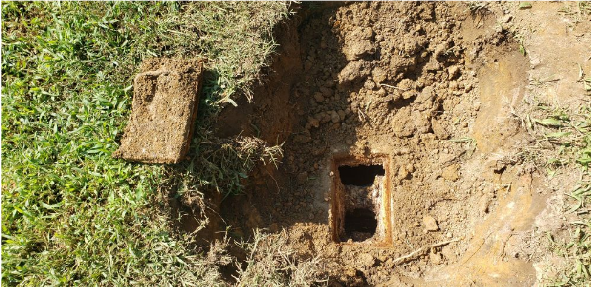
View of Septic Tank Outlet End
