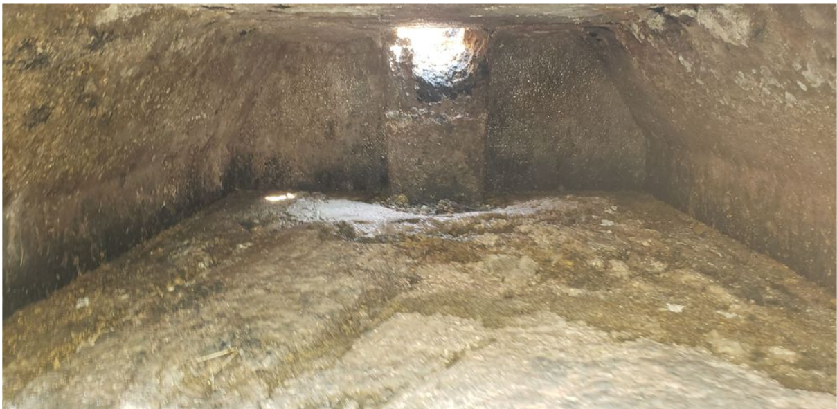
View of Inlet Compartment After Pumping of Tank
