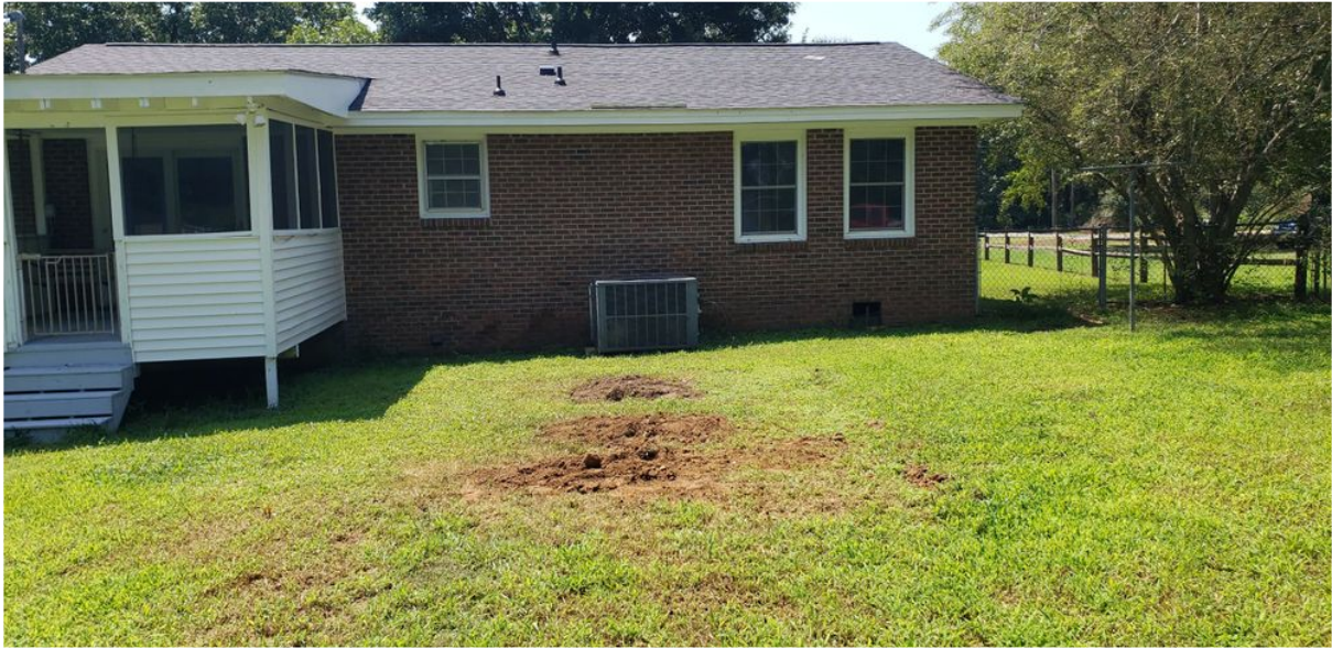
Excavations Filled and Site Cleaned
