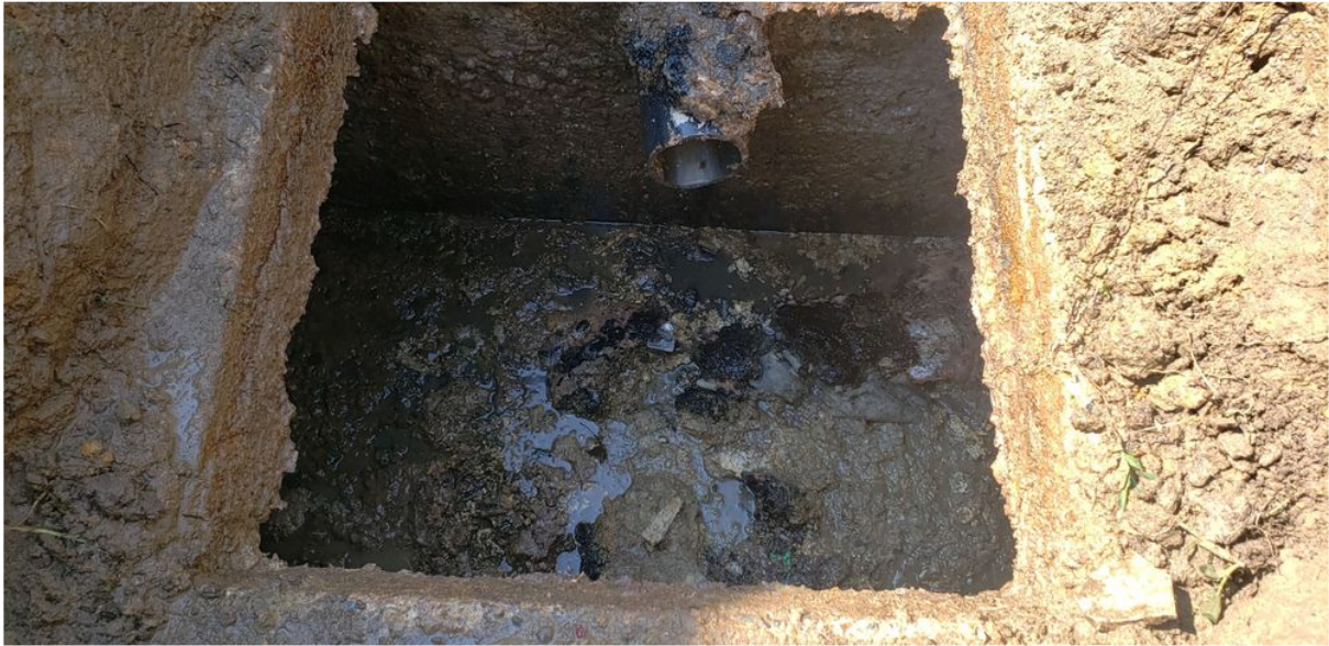
View of Septic Tank Inlet End
