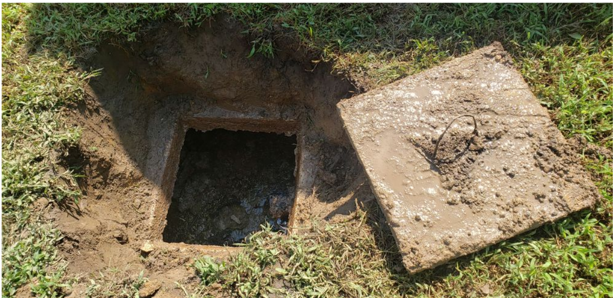
View of Septic Tank Inlet End
