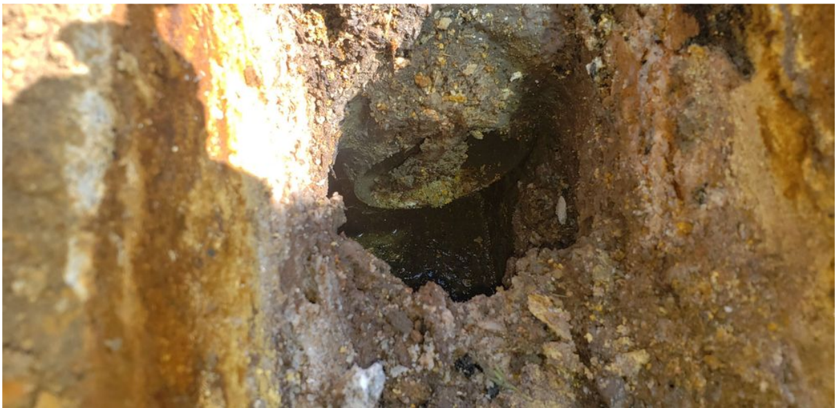
View of Septic Tank Outlet Tee
