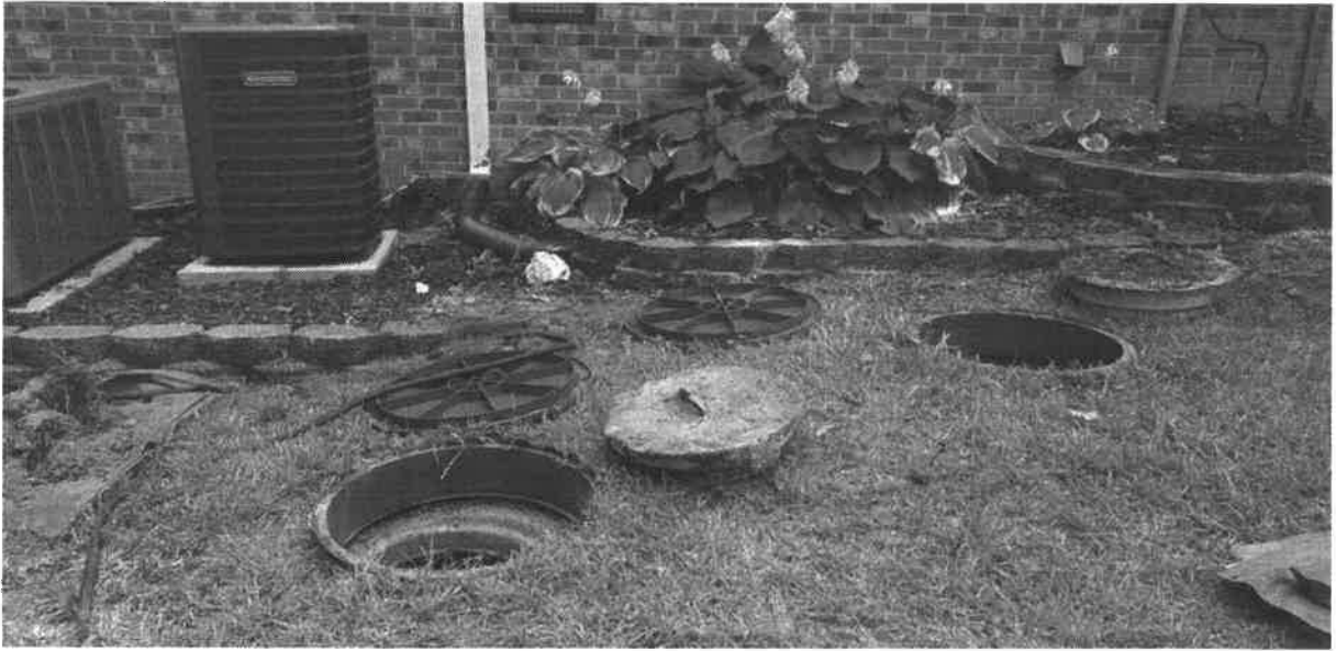
View of Location of Septic Tank Inlet and Outlet Lids
