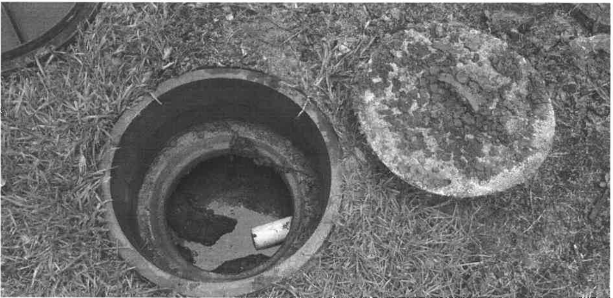
View of Septic Tank Inlet End
