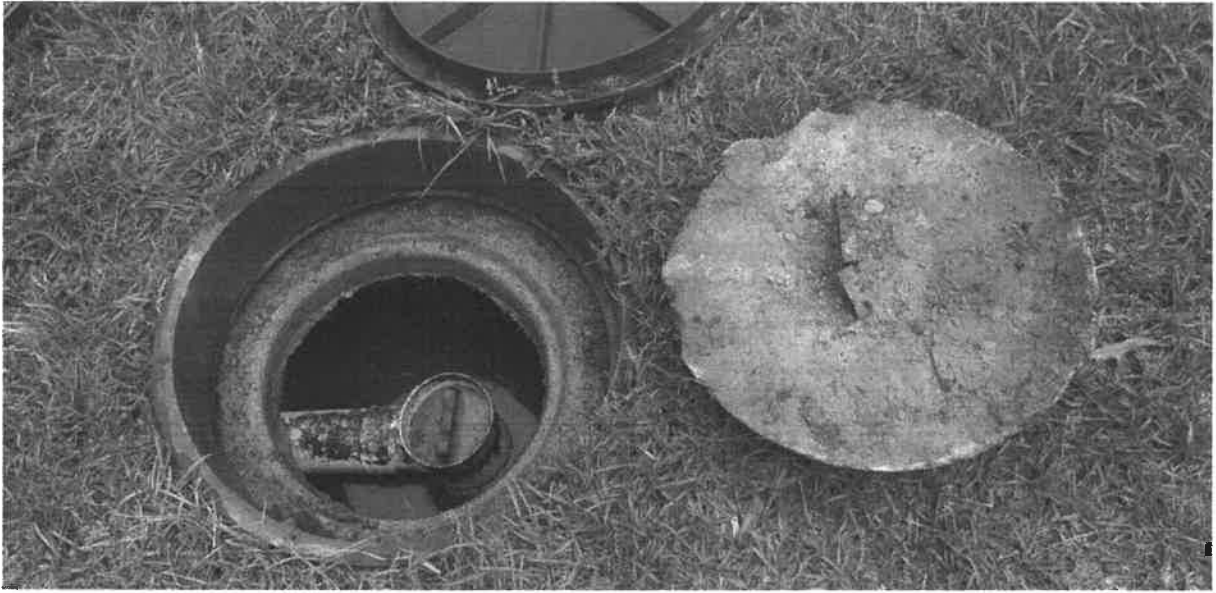
View of Septic Tank Outlet End
