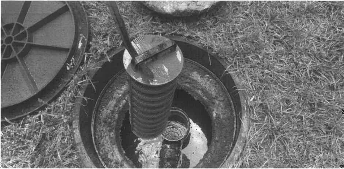
View of Clean Outlet Tee Filter
