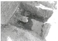
The distribution box is deteriorated/ damaged. The integrity of the box is compromised, and replacement is needed. Contact a repair professional about replacing the D-Box.
