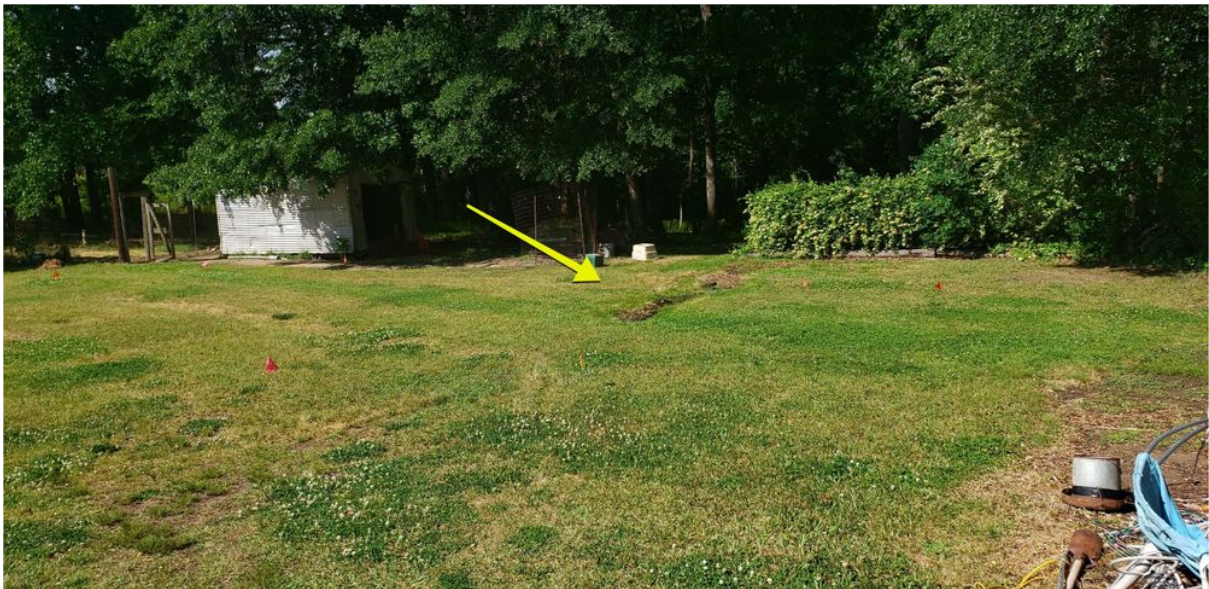
Area of Surfacing Effluent
