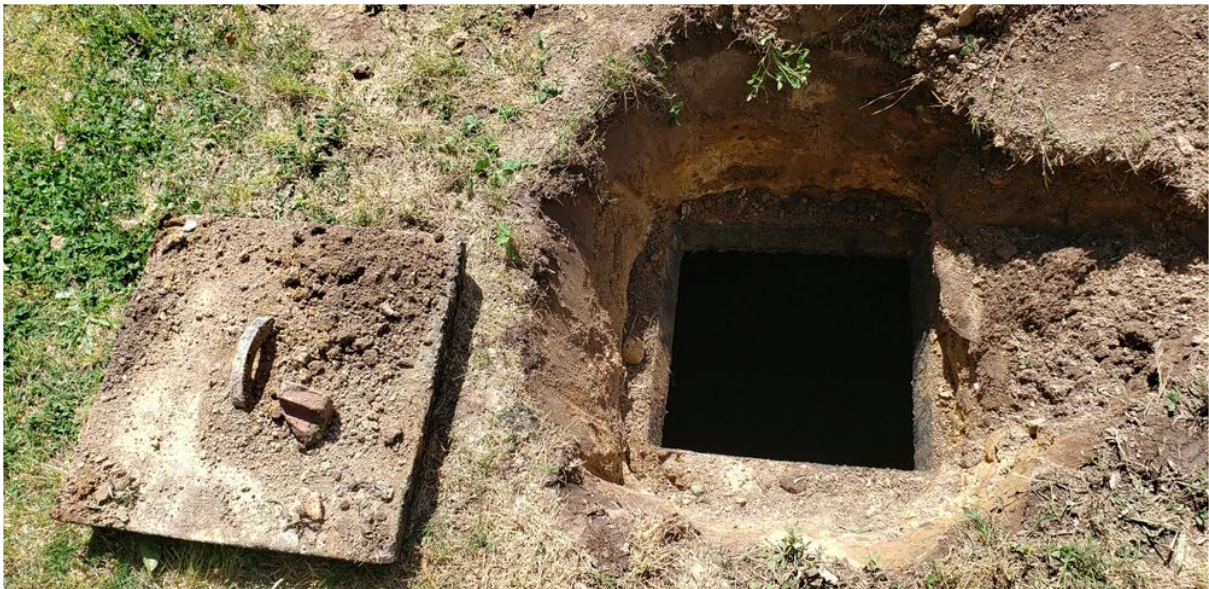
View of Septic Tank Inlet End
