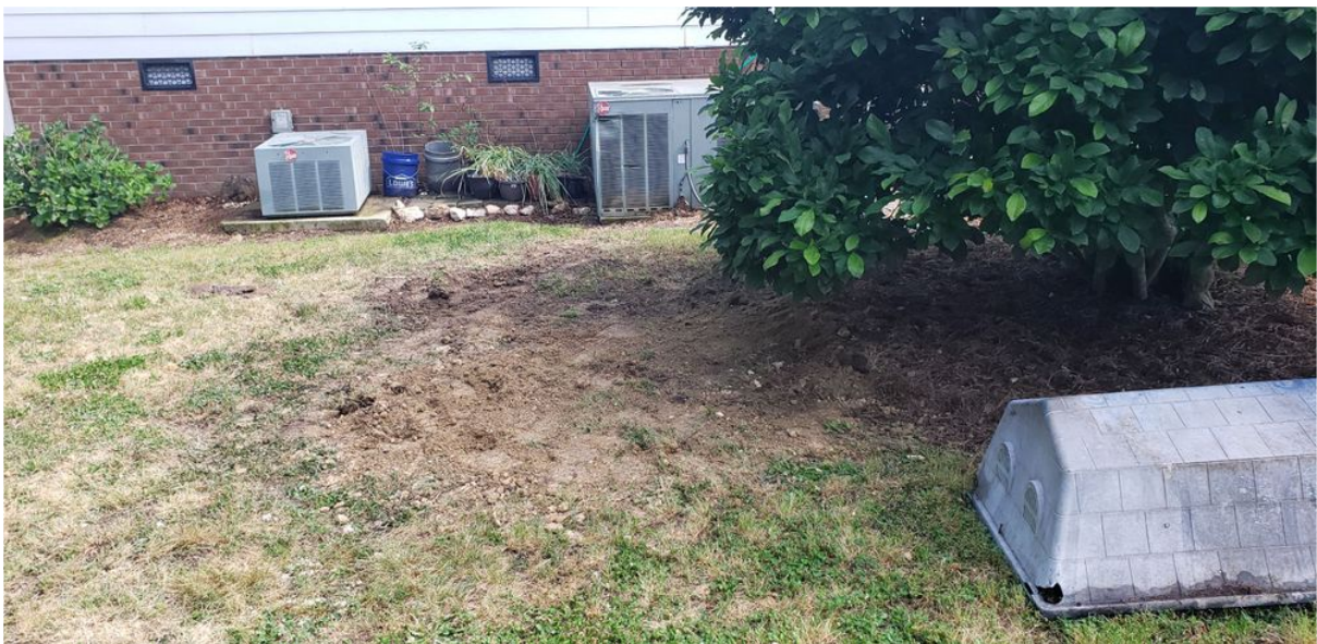
Excavations Filled and Site Cleaned
