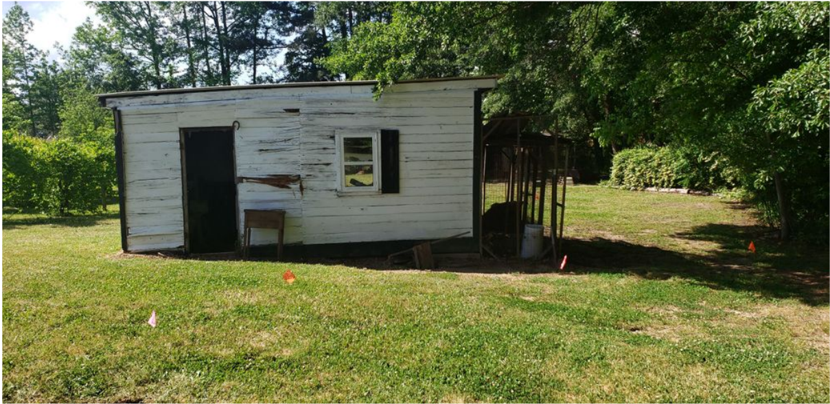
View of Storage Shed Over Dispersal Field
