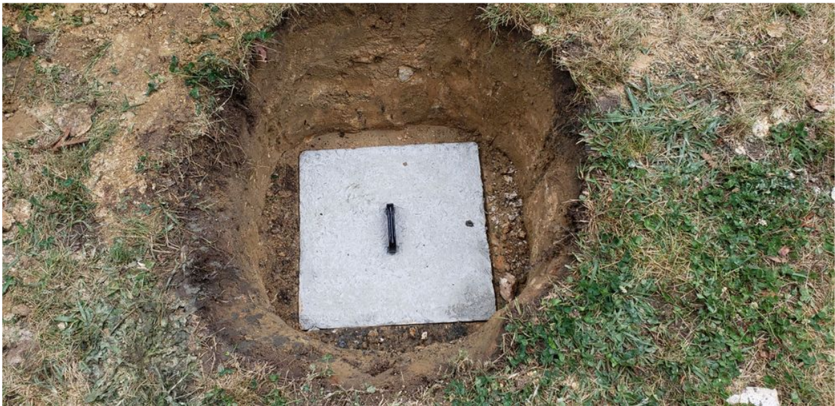
View of Replacement Outlet Lid Placed By Inspector
