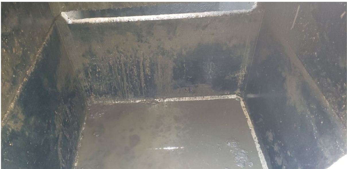
View of Septic Tank Inlet Compartment After Pumping Tank
