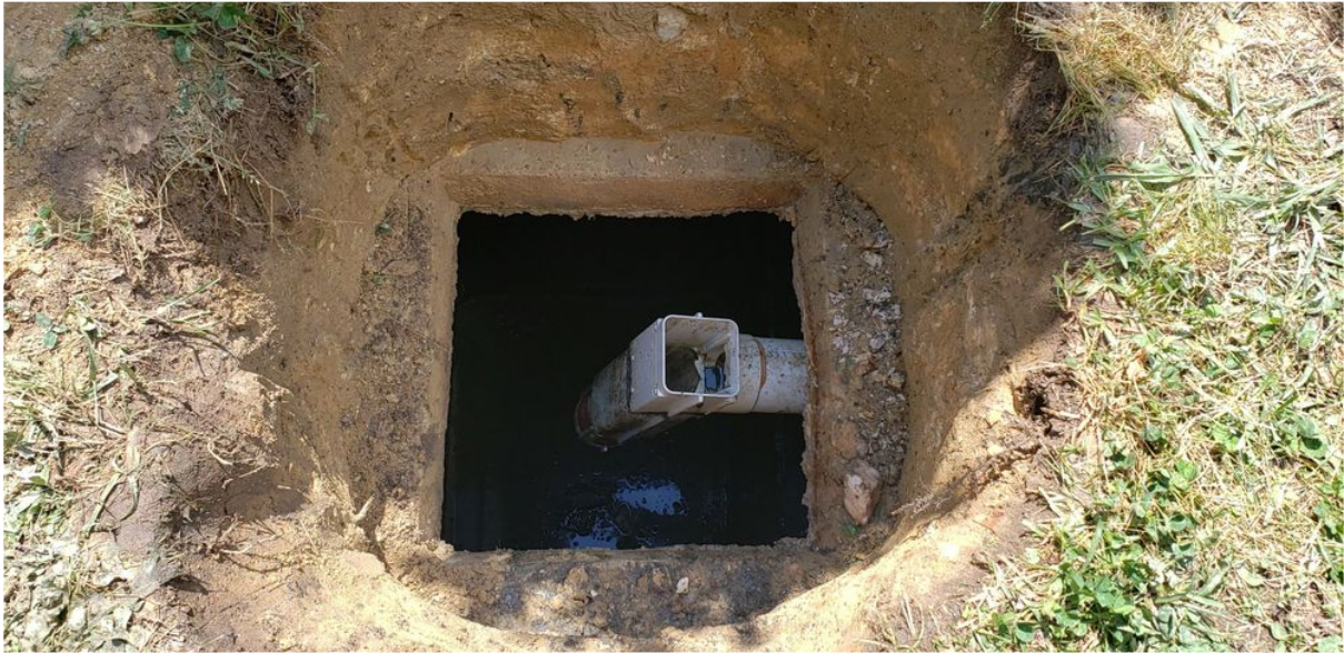
View of Septic Tank Outlet End
