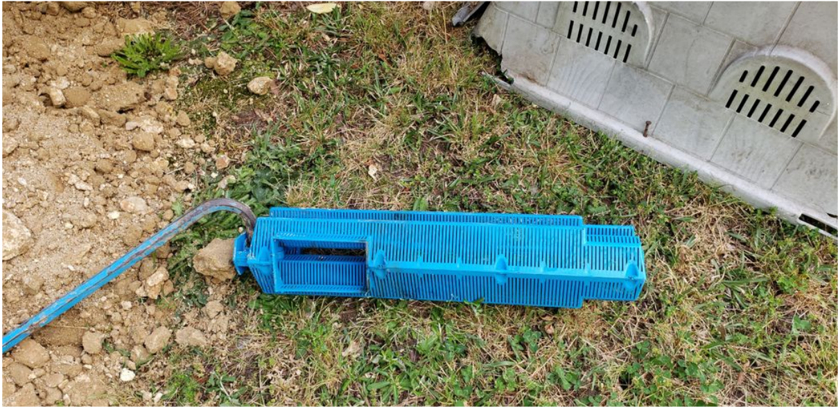
View of Cleaned Outlet Tee Filter
